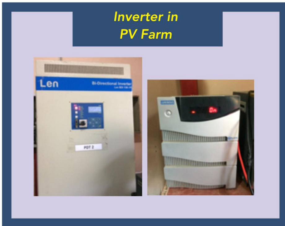
Gambar 35. Bi-Directional Inverter
