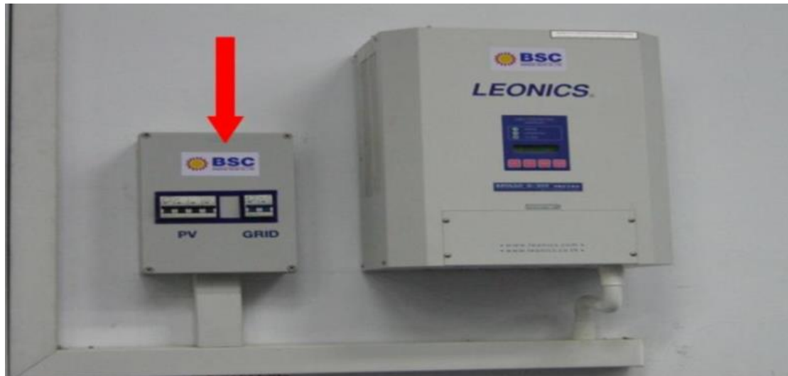
Gambar 39. Disconnecting Switch DC Side dan AC Side
