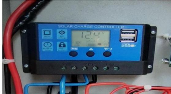
Gambar 20. Solar Charge Controller PWM 30A
