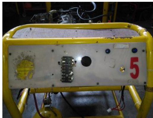
Gambar 38. Kondisi Awal Board Panel
