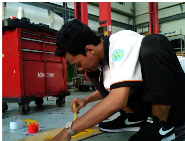
Gambar 70. Proses pengecatan garis penanda
