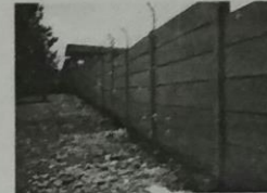
Dinding Batu Beton
