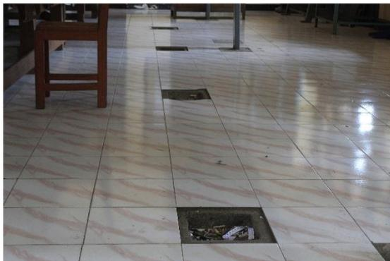
Gambar 15. Lubang Grounding
