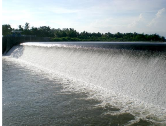
Gambar 2. Bendungan Tegay, Kali Opak, Imogiri
