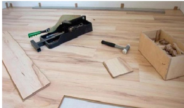
Gambar 2. Pekerjaan finishing kering pasang parket
