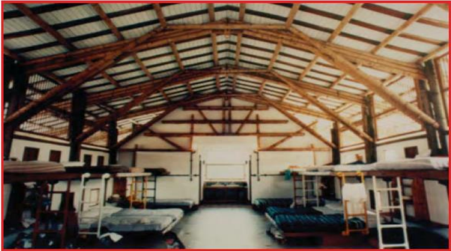
Gambar XI-40, Rangka Atap Bambu
