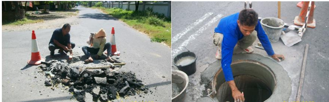
Gambar 7. Peninggian Manhole Jaringan Sumber: Balai IPAL Sewon, 2014
